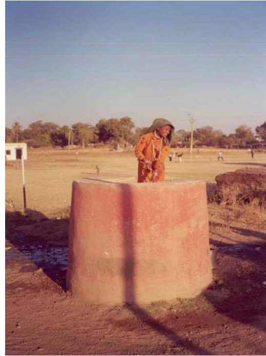
Villagers use these Air Shafts like wells as water flows through the tunnels throughout the year
