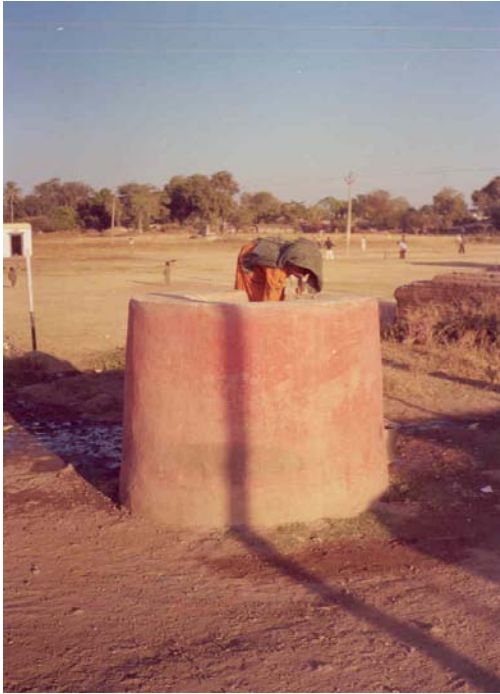
Villagers use these Air Shafts like wells as water flows through the tunnels throughout the year
