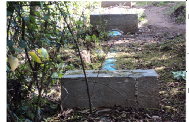
Laying of Clear Water Rising Main comprising of 300mm \phi D.I. Pipes in progress.
