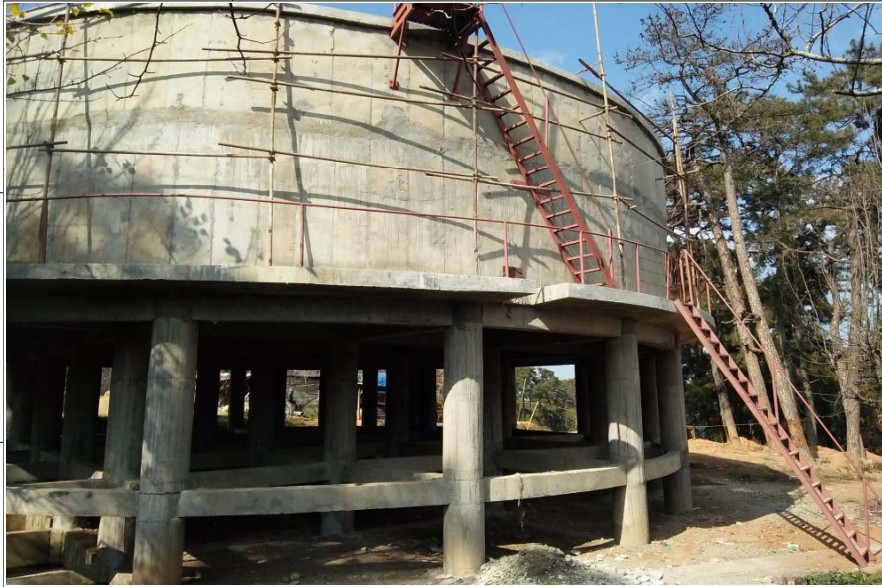
Zonal Reservoir of 1.12ML capacity with 3.00m staging for Laitumkhrach area with location at Fruit Garden is completed.
