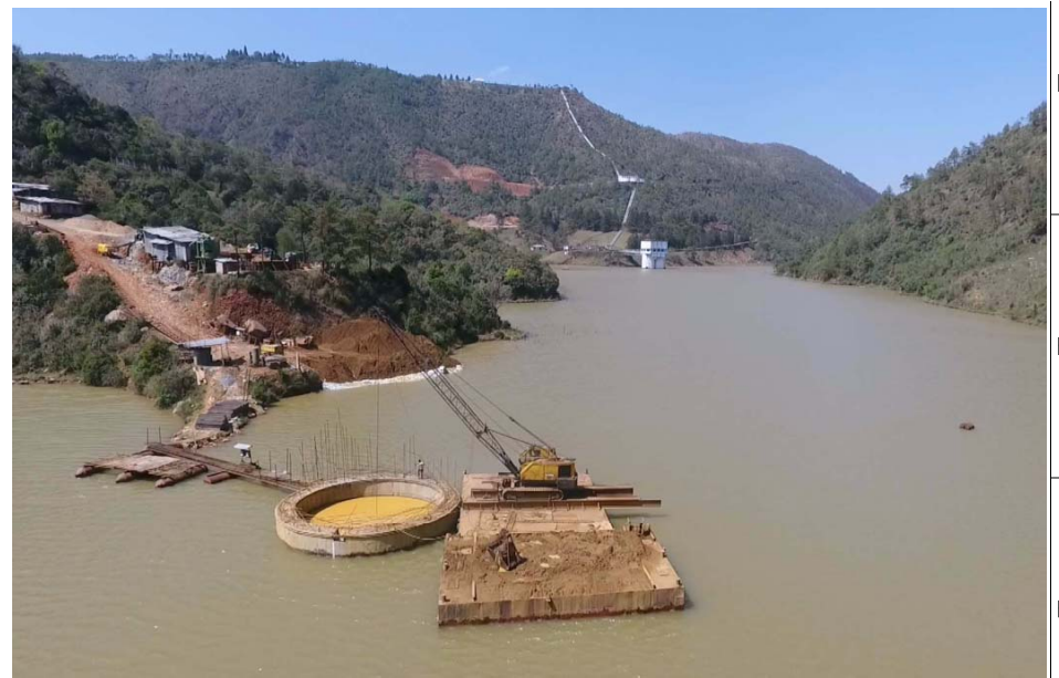
Construction of RCC Intake Well is in progress.
