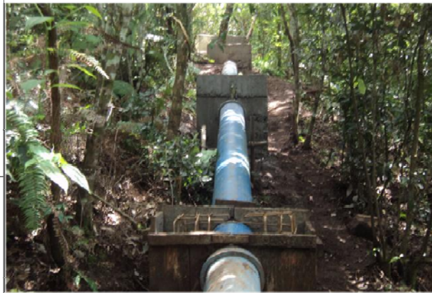
Laying of Clear Water Rising Main comprising of 300mm \phi D.I. Pipes in progress.
