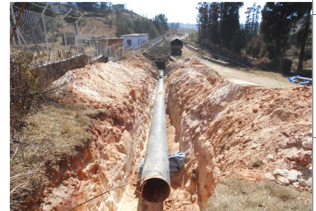
Laying of Raw Water Rising Main comprising of 508mm \phi M.S. Pipe in the process.
