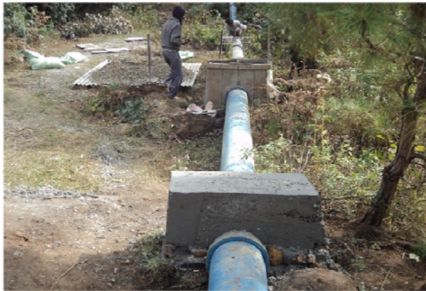
Laying of Clear Water Rising Main comprising of 300mm \phi D.I. Pipes in progress.
