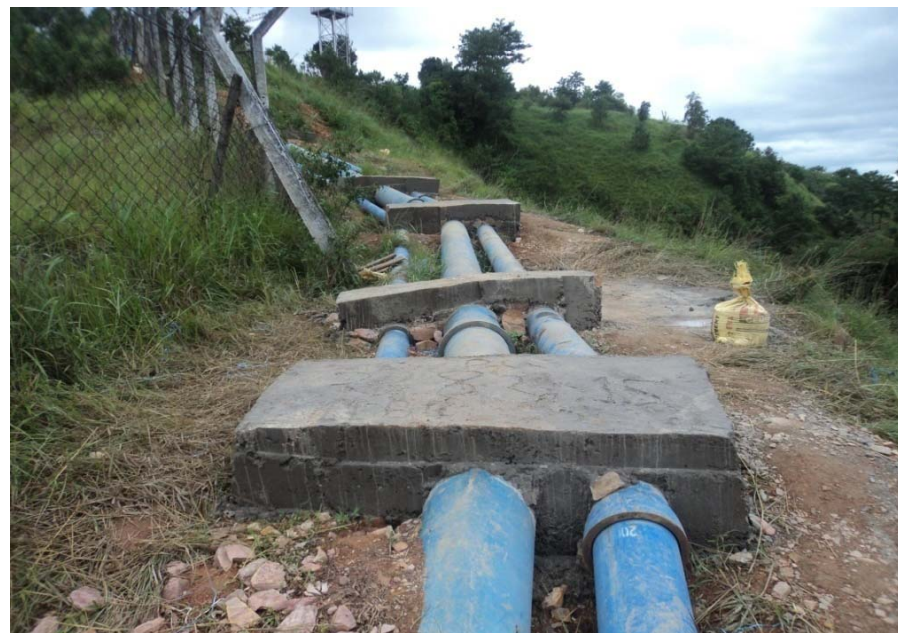
Laying of Clear Water Gravity Main from 6½ Mile comprising of 300mm, 200mm & 150mm D.I. Pipes for Nongmynsong, Cantonment Board and Mawlai respectively, in progress.
