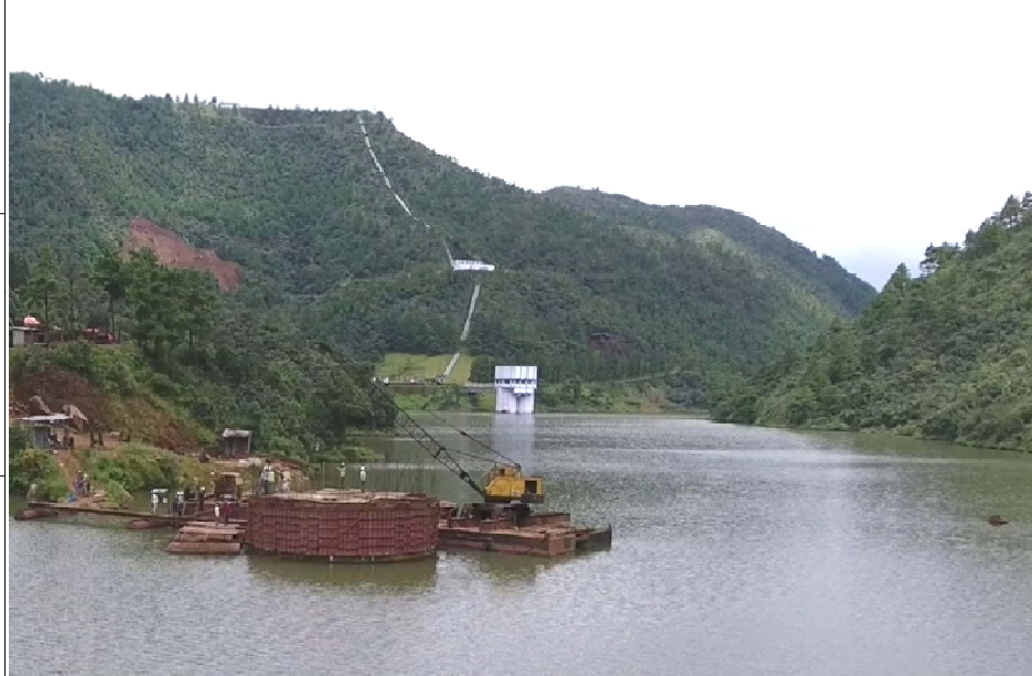
Construction of RCC Intake Well is in progress.
