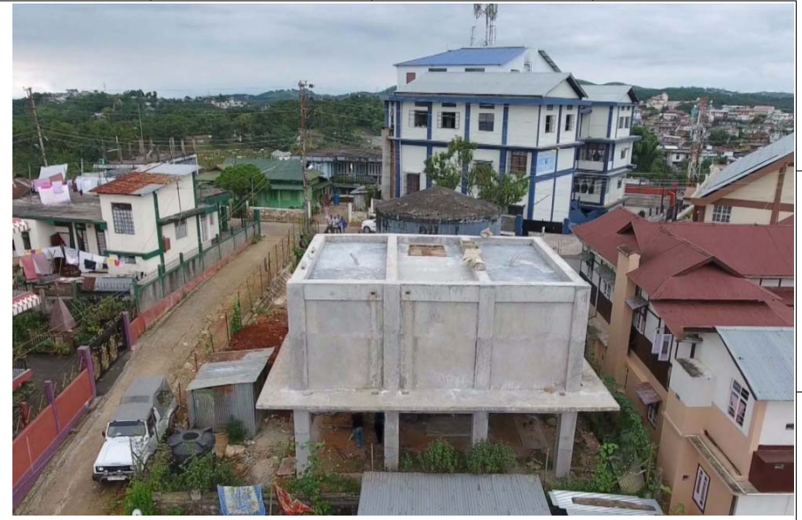
Zonal Reservoir of capacity 0.14 ML with 3m Staging for Mawlai area with location at Mawlai Nongkwar is completed
