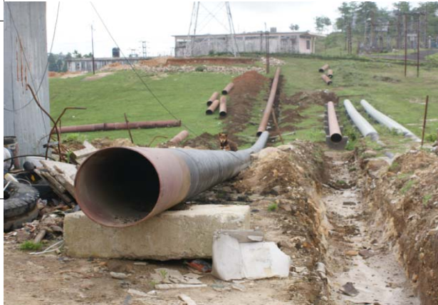
Laying of Raw Water Rising Main comprising of 508mm \phi M.S. Pipe in the process.
