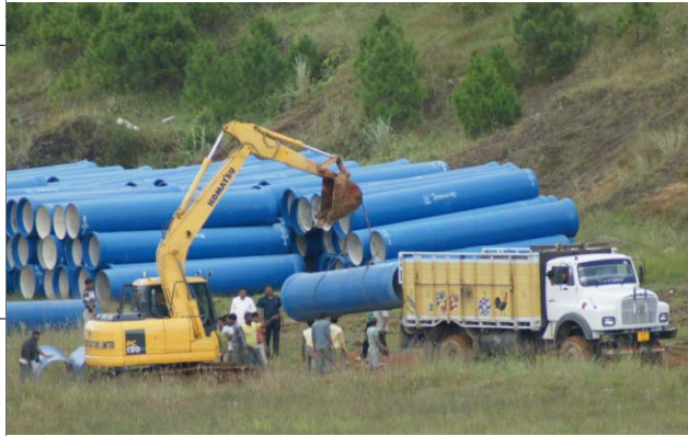
Transportation and Laying Gravity Main comprising of 1000/900/750 mm \phi DI pipes
