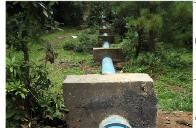
Laying of Clear Water Rising Main comprising of 300mm \phi D.I. Pipes in progress.
