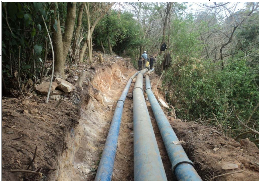
Laying of Clear Water Gravity Main from 6½ Mile comprising of 300mm, 200mm & 150mm D.I. Pipes for Nongmynsong, Cantonment Board and Mawlai respectively, in progress.
