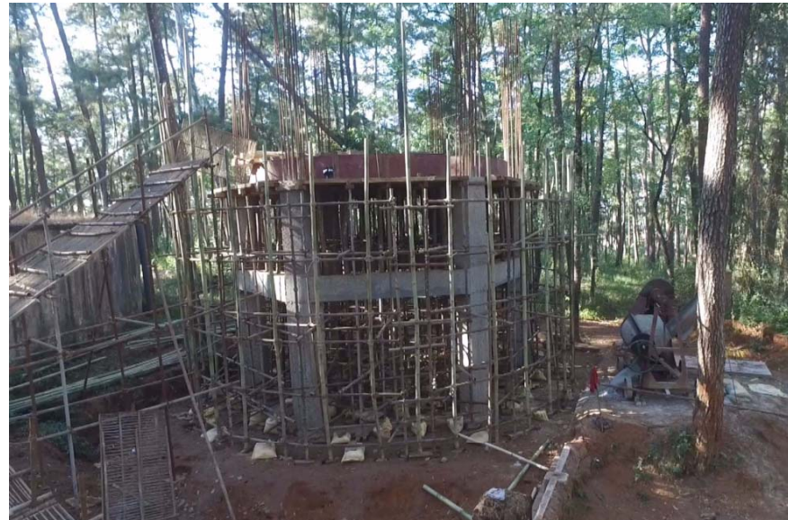
Zonal Reservoir of capacity 0.09 ML with 6m Staging for Mawlai area at Mawlai Mawroh is in progress
