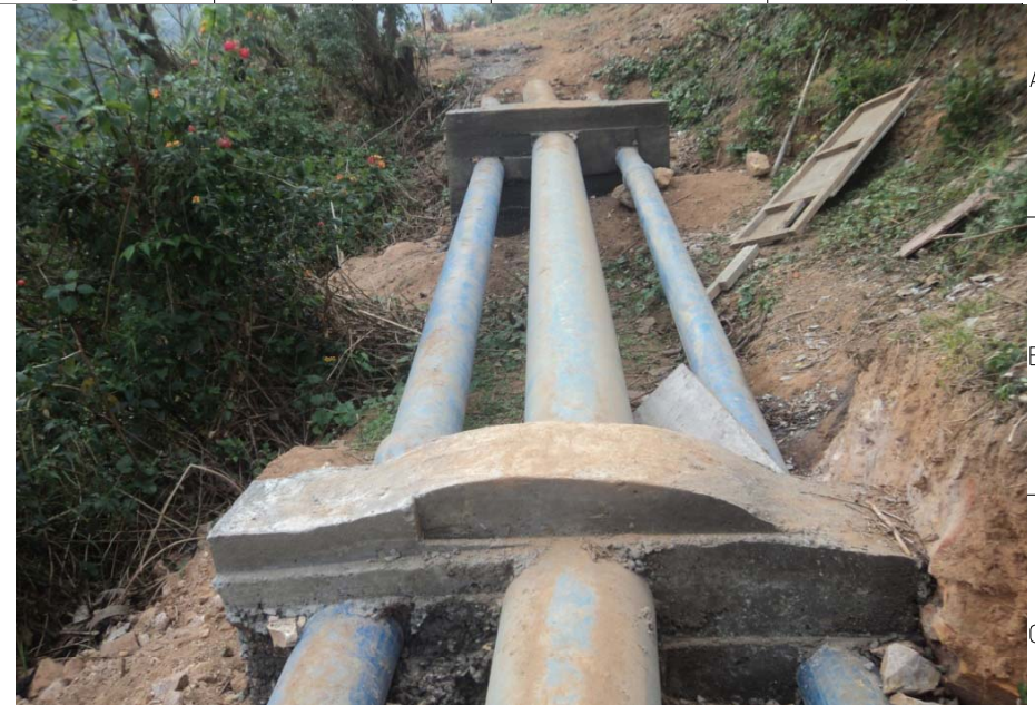
Laying of Clear Water Gravity Main from 6½ Mile comprising of 300mm, 200mm & 150mm D.I. Pipes for Nongmynsong, Cantonment Board and Mawlai respectively, in progress.
