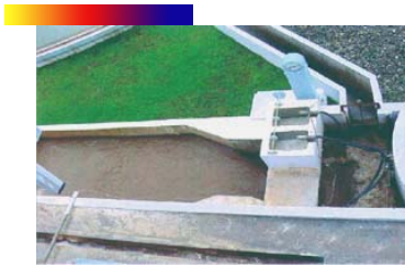
Raw water is received at the Inlet to Treatment Plant
